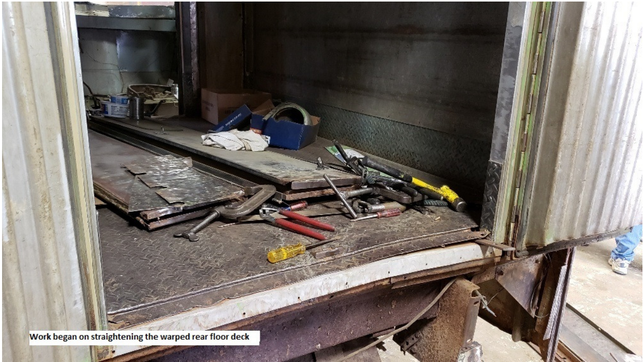
Work began on straightening the warped rear floor deck
